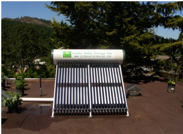
Residential Installation in Victoria, BC
