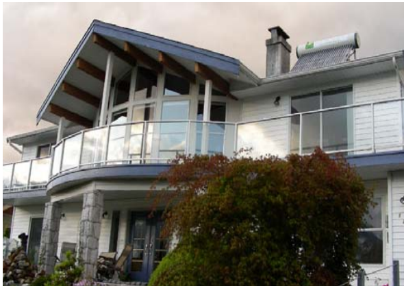
Residential Installation in Squamish, BC
